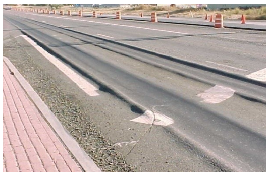
Figure 2.14A Pictorial View of Rutting
