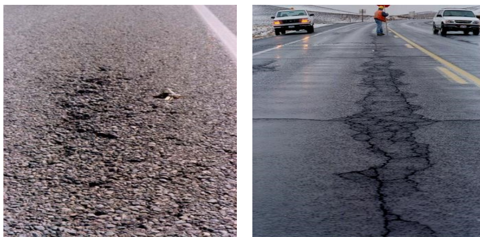
Figure 2.11 A Pictorial View of Raveling
